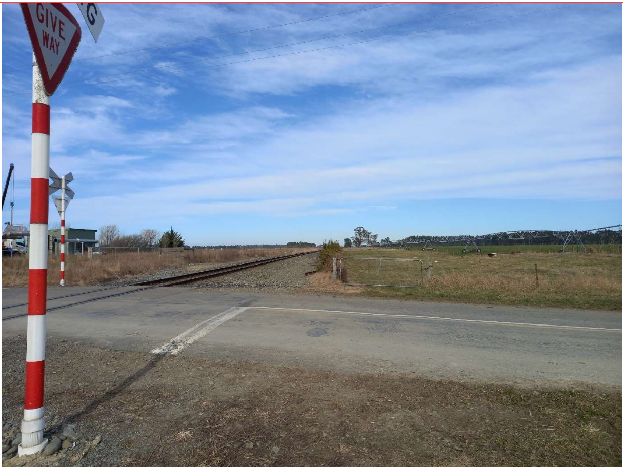
Figure 14: West Approach – looking south (Down Track) from 1.5m back from limit line
