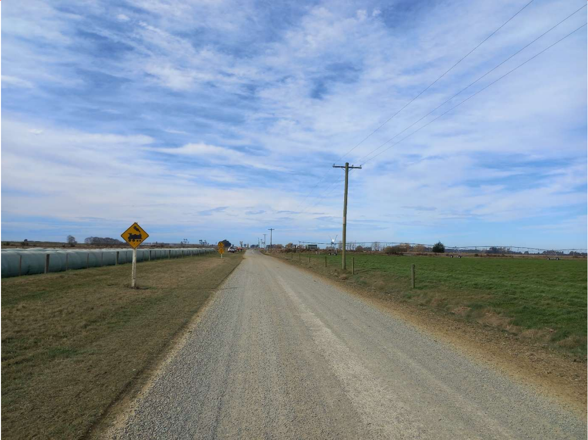
Figure 12: West Approach Carrolls Road – looking east from Outer Advanced Warning Sign
