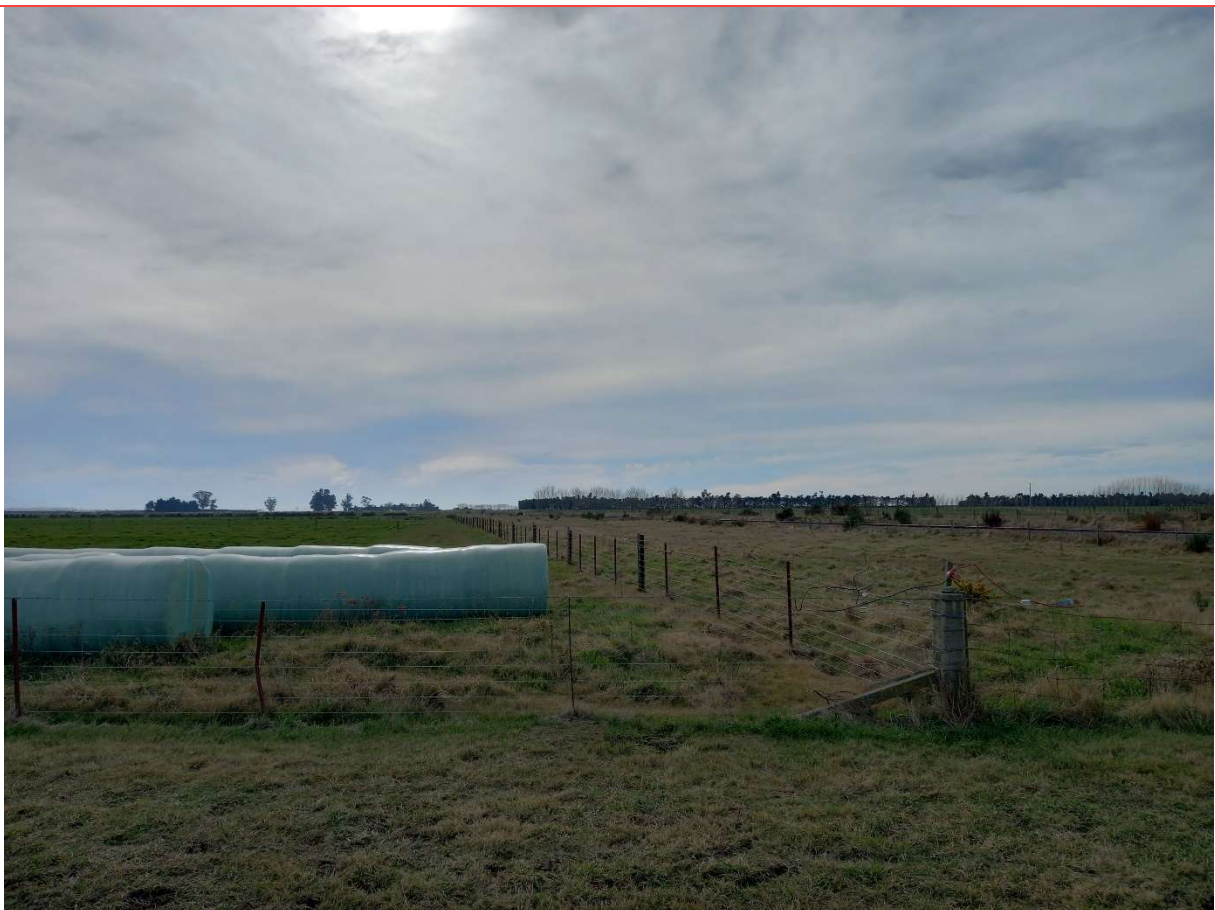
Figure 15: West Approach – looking east from 35m back from limit line
