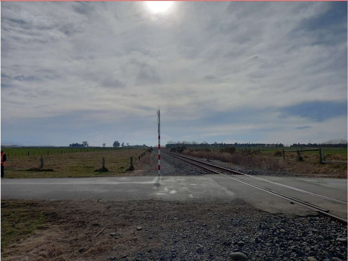
Figure 9: Looking North (Up Track)
