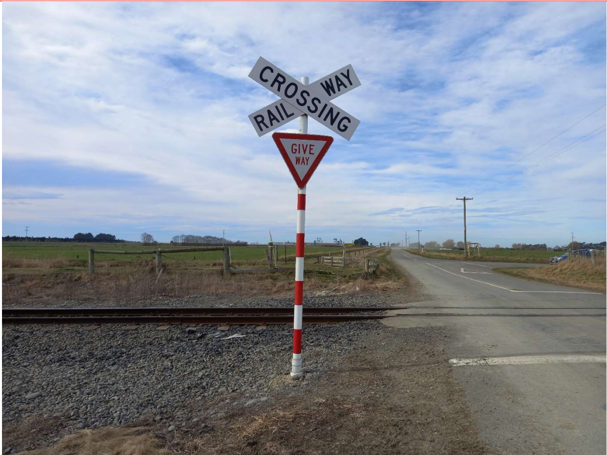
Figure 16: West Approach – RPX-3 Signage
