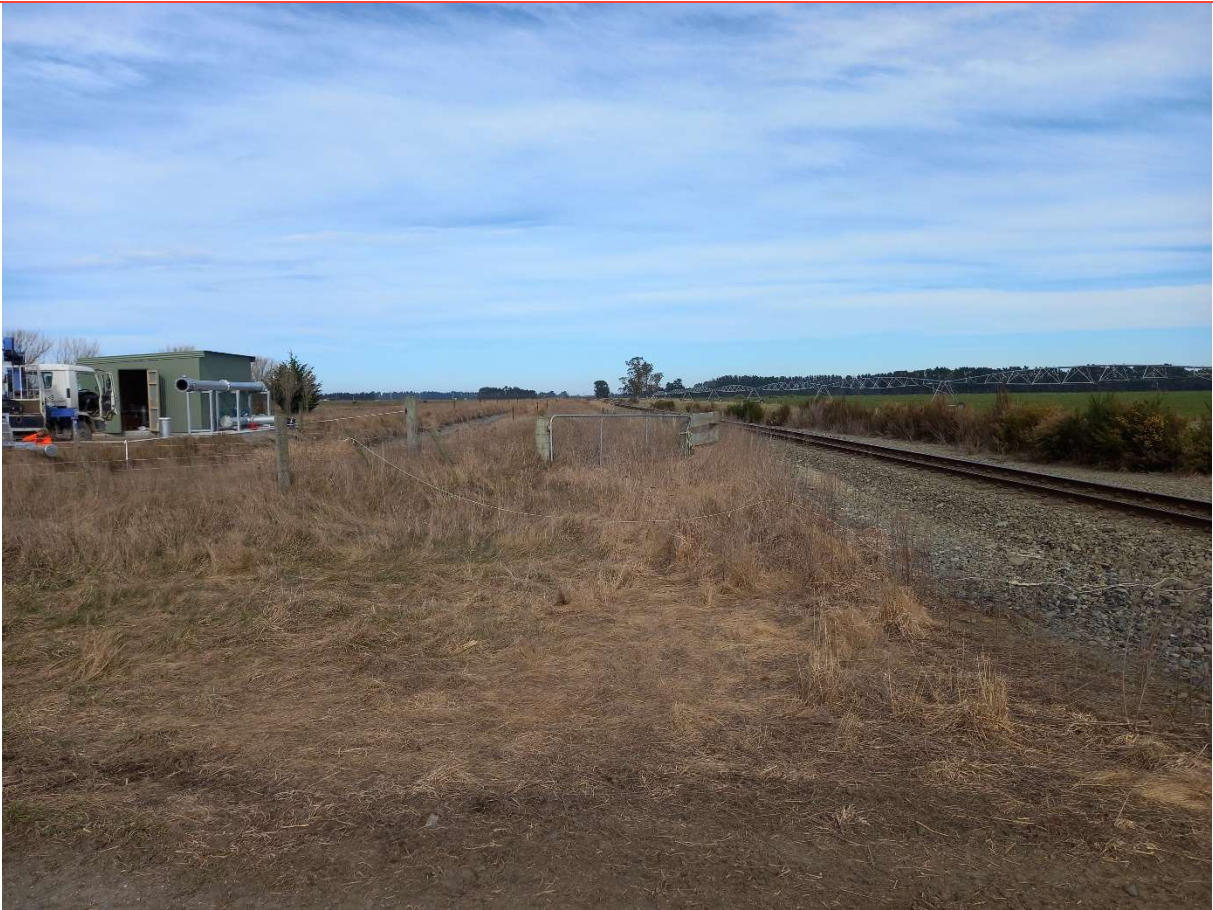
Figure 7: East Approach – looking south (Down Track) from 1.5m back from limit line
