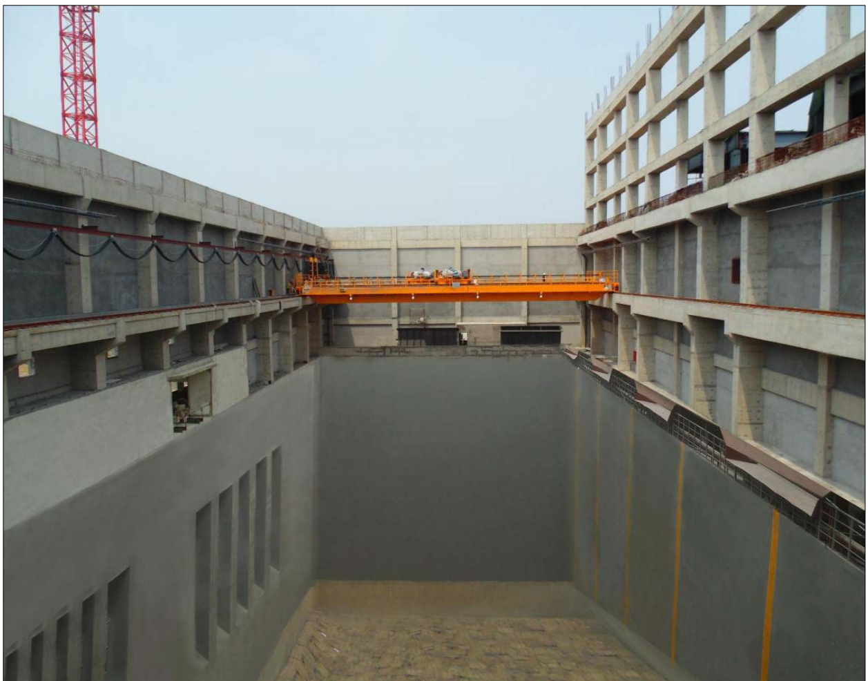
Figure 39: Waste bunker under construction
