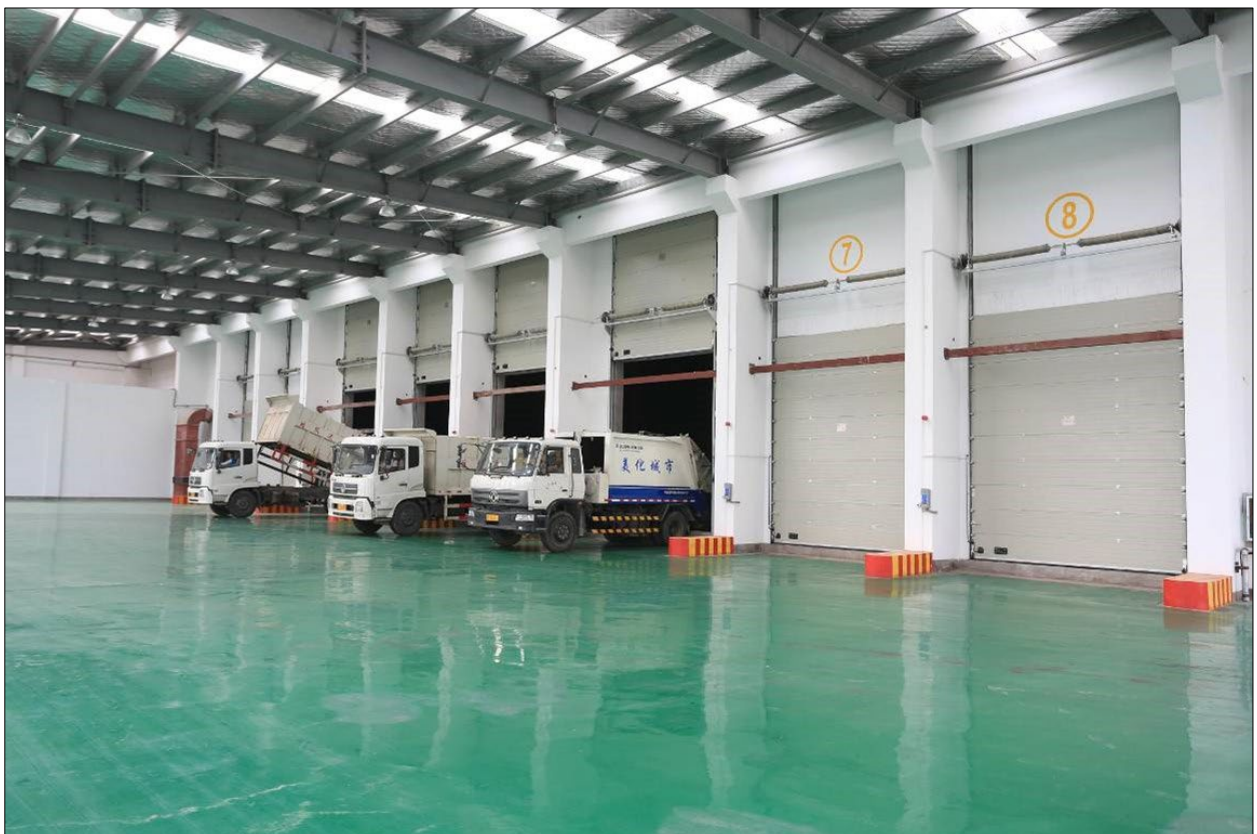
Figure 7: Trucks in the unloading hall tipping waste directly into the waste bunker beyond.
