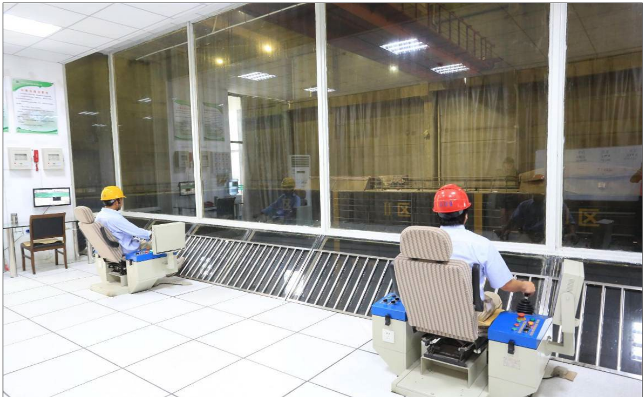
Figure 13: Grapple crane operators at work with a view over the waste bunker.
