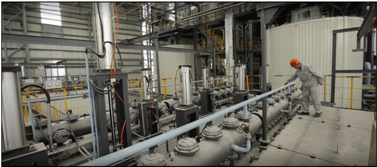
Figure 22: Top of baghouse showing pulse jet cleaning system and chamber isolation valves.
